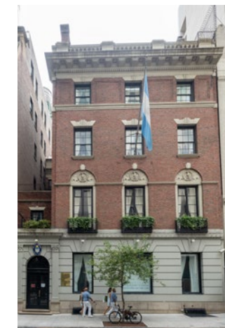
12 WEST 56 TH ST HARRY B. HOLLINS RESIDENCE
