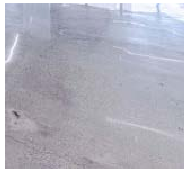
POLISHED CONCRETE FLOOR FLOORING
