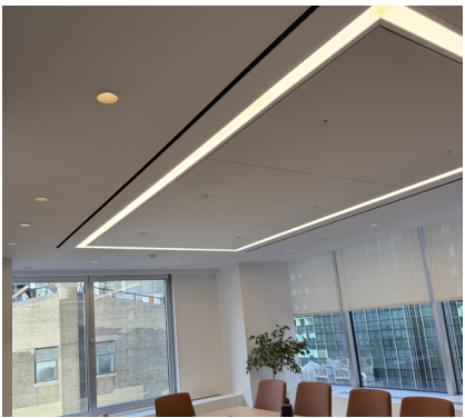
BOARDROOM CEILING Sheetrock surround with Act tile and rectangular light fixture
